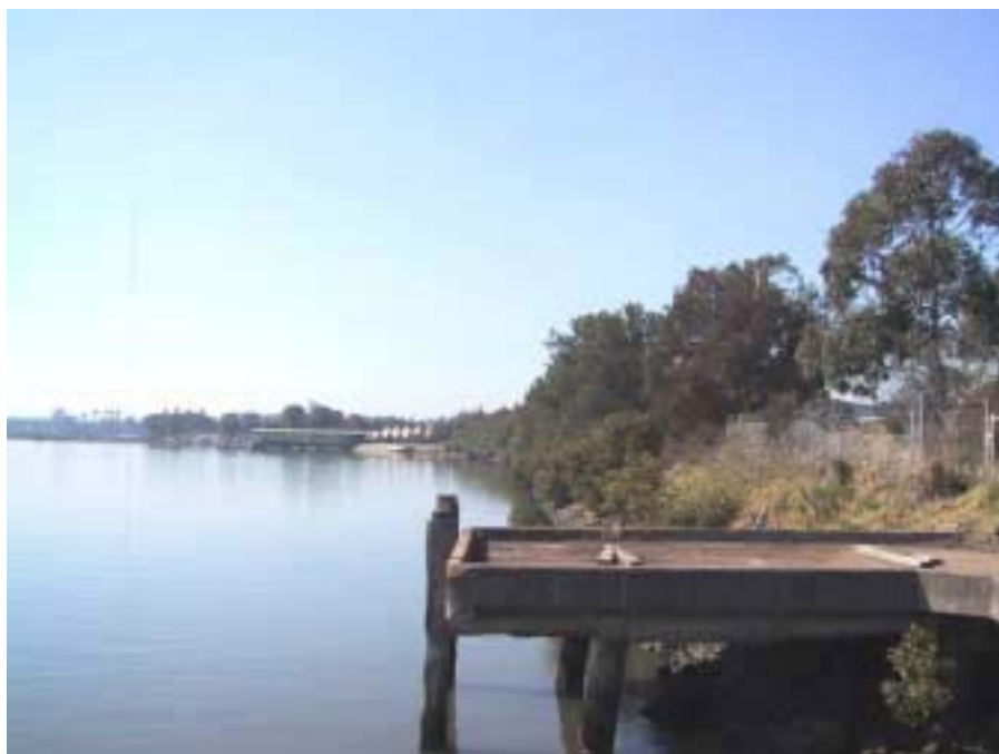
Figure 1. The Parramatta River Frontage.
