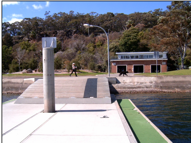
Figure 5.3 Water access structure, Pearl Bay, Mosman
