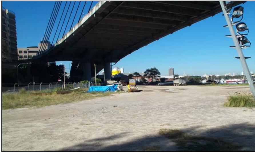
Figure 2.1: Photos of the existing site
