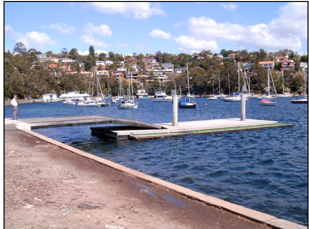
Figure 5.4 Water access structure, Pearl Bay, Mosman
