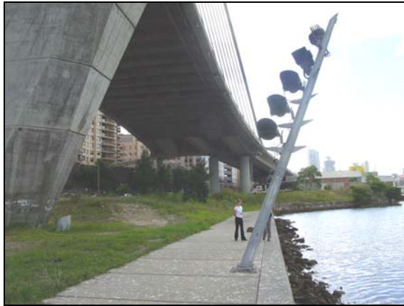
Figure 4.1: Existing paving at NSW Maritime site, April 2004
