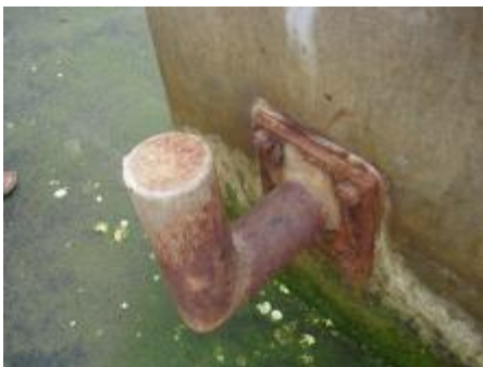
Corroded mooring cleat and bollard.
