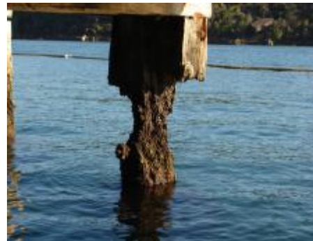
Examples of piles and necking (hour-glass shape)
