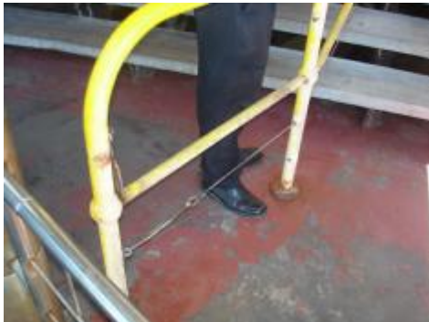
Corroded connections at the base of the handrail.
