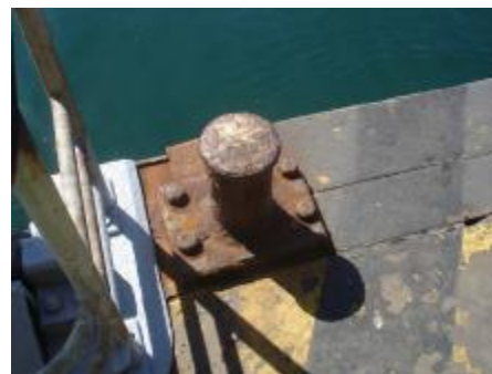
Corroded mooring cleat and bollard.
