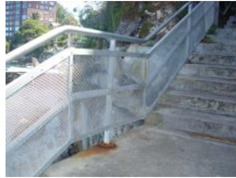
Corroded connections at the base of the handrail.
