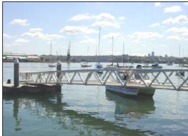
Example of an Access Ramp ( gangway )
