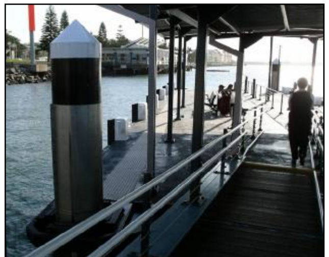
Example of handrailing
