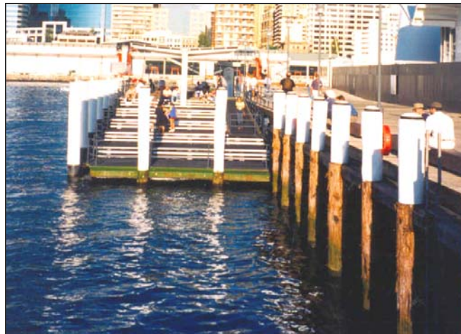
Example of a Fixed Wharf structure
