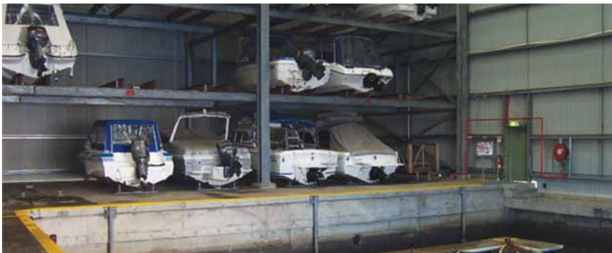
Figure 7: dry stack storage facility
